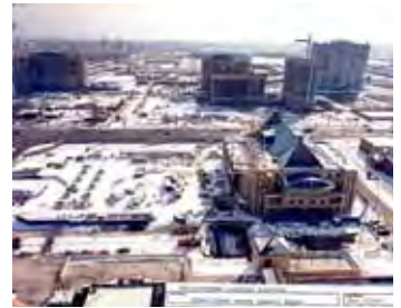
Library under construction, January 1990, Canadiana Room, MLS
